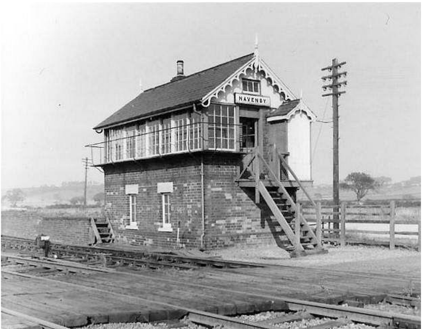
Navenby Signal box located between the southbound platform and the goods shed.
